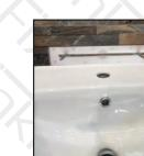
6. Offer up the basin to the protruding bolts and insert the nylon bushings through the wash basin holes (shown opposite). Screw on the flange nuts. Adjust the bushings to obtain the correct level then holding the 'wings', tighten the flange nuts using a 15mm spanner.
